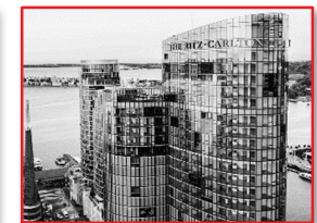
▶ Formwork and Facades
