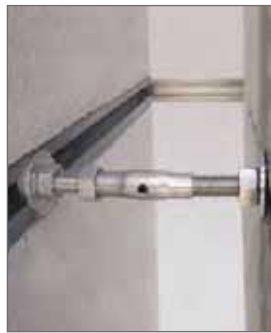
Turnbuckle Connections JSV provide three-dimensional alignment.
