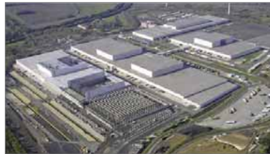
Installed on roof.
