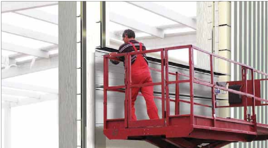
Installation of a multi-layer insulated profiled metal sheet wall.
