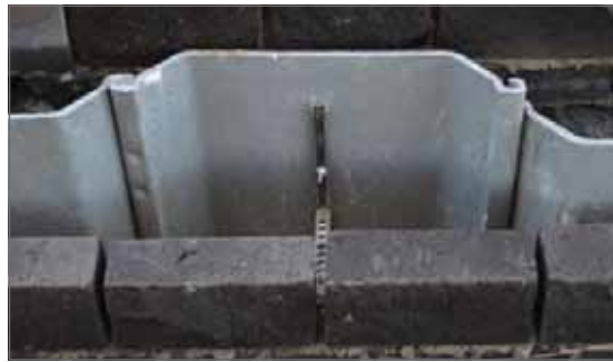
Connection of brickwork to sheet-pile wall.
